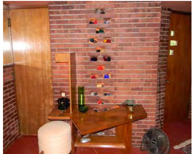
Note how the stones are included in brick
